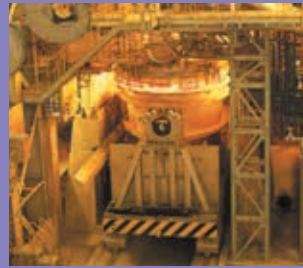
取鍋精錬設備 Ladle furnace
