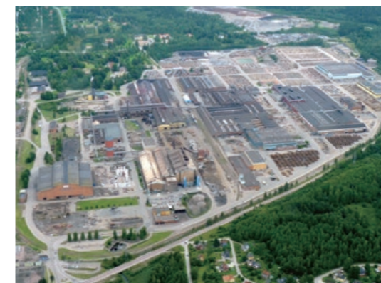
Hofors mill of Ovako, where the hydrogen plant is being constructed
