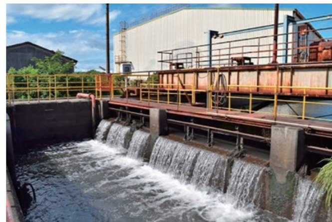
Wastewater treatment facility
