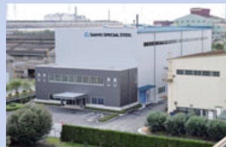
The No.2 metal powder plant
