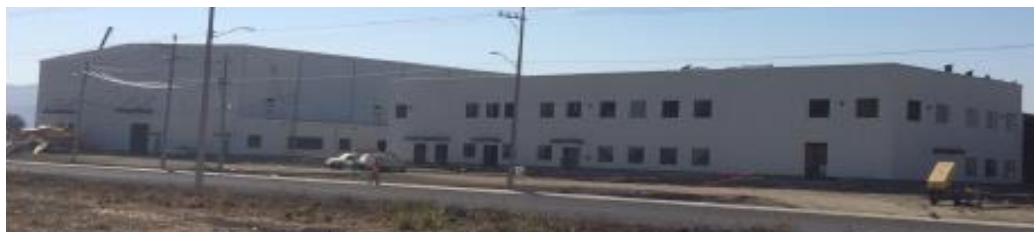
< Plant under construction >
