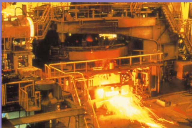
150t UHP電気炉 150-t UHP electric arc furnace
