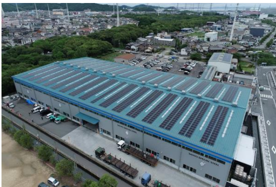
Photovoltaics installed on the roofs of product warehouse
